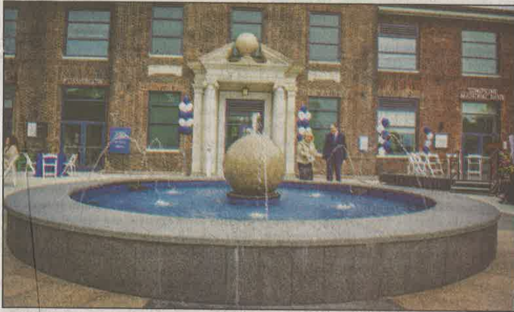
A renovated and nearly filled Boyce Thompson property in Executive Park Yonkers.
